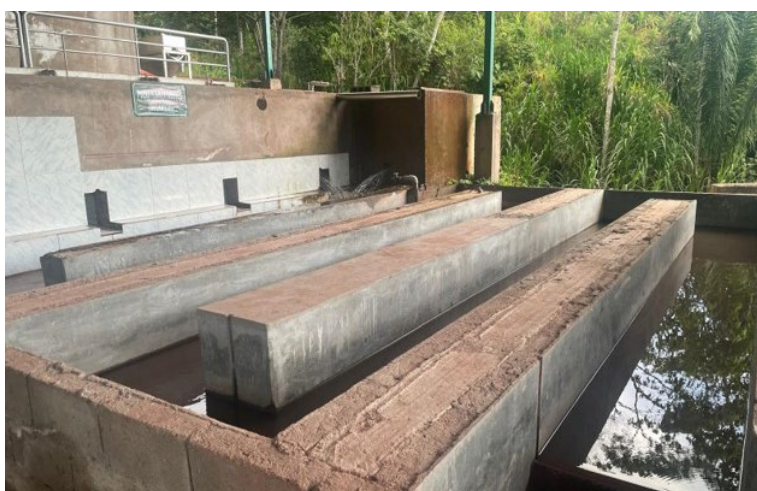
Fermentation and washing tanks used in coffee processing. Source: ICF
