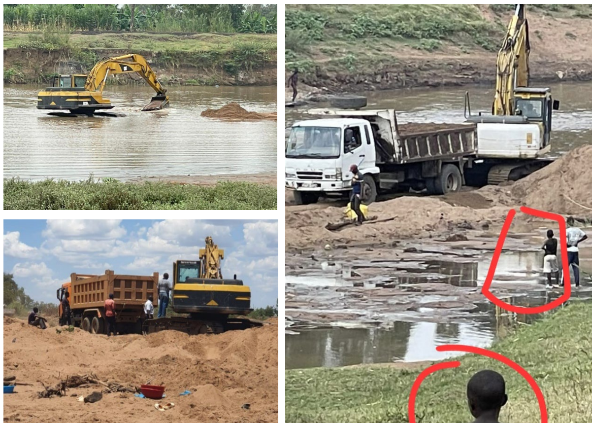
Figure 4. Excavators loading sand near Kuja River in Homa Bay County
