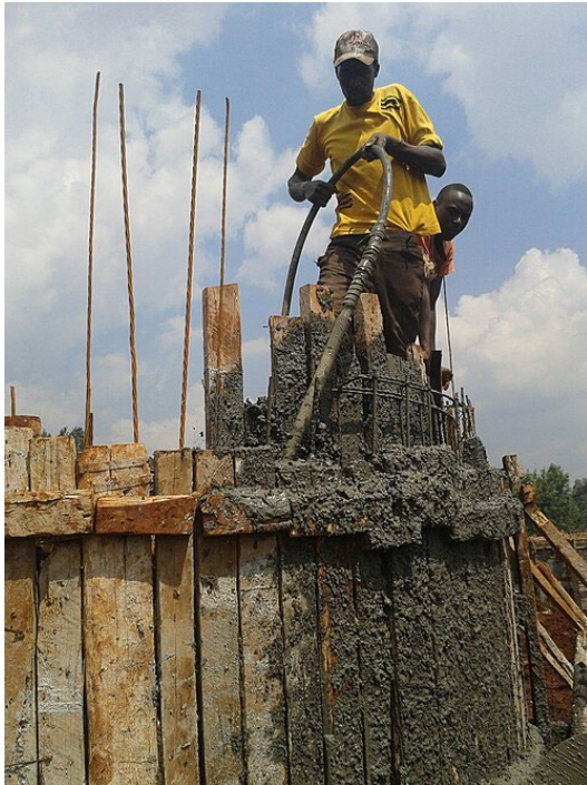
Figure 17. Pouring concrete
