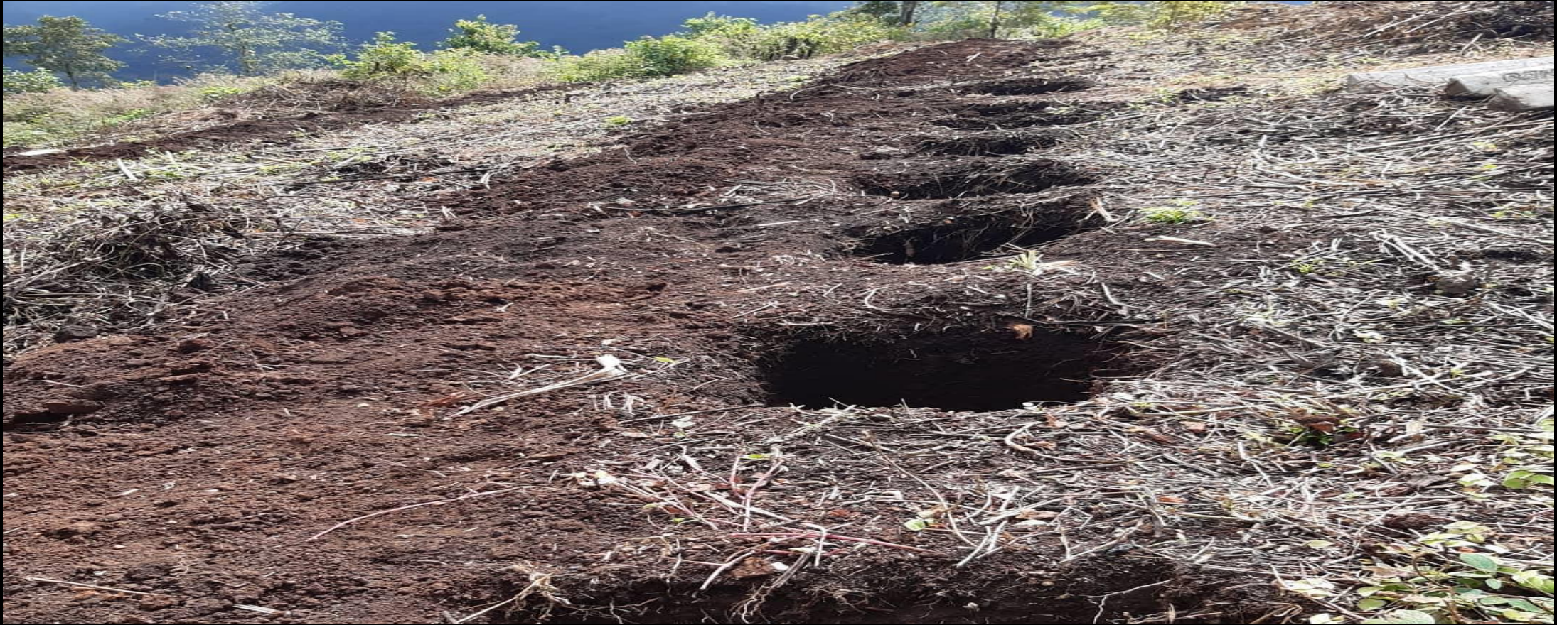
Blocking and digging of canal
